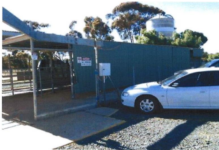
Skillion workshop facility
