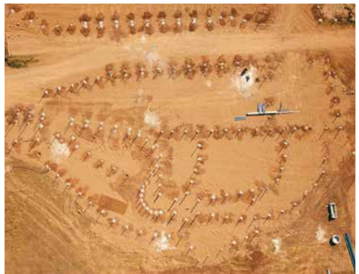
Cementing in the posts for the "Cregmore Yards."
